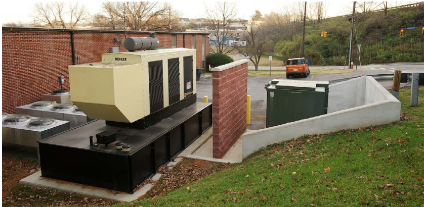
New emergency generator, pad-mounted transformer, and firewall
